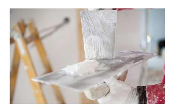
• Graphenstone® MortarBase Premium is a natural bed mortar with graphene technology suitable for rendering, grouting on rehabilitation works, in addition to restoration processes of buildings. The product has coarse aggregate, so it is applied as first regulation coat and can be used in most common construction surfaces, as brick, concrete or masonry.
