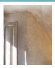
• Graphenstone® Firenzza is a natural hydraulic lime mortar with graphene technology highly flexible and tough, which is suitable for the performing of high-end decoration structures. The product is used for rendering and plastering, and its application provides a mineral finishing with a significant breathability and durability.
