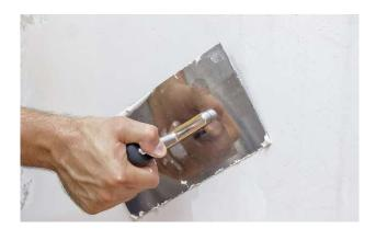
• Graphenstone® Naturglue Premium is an ecological adhesive mortar with graphene technology which is characterized by its high quality and flexibility. The product is suitable for bonding ceramic tiles, as well as for anchoring procedures of insulation boards and non-flooding solutions.
