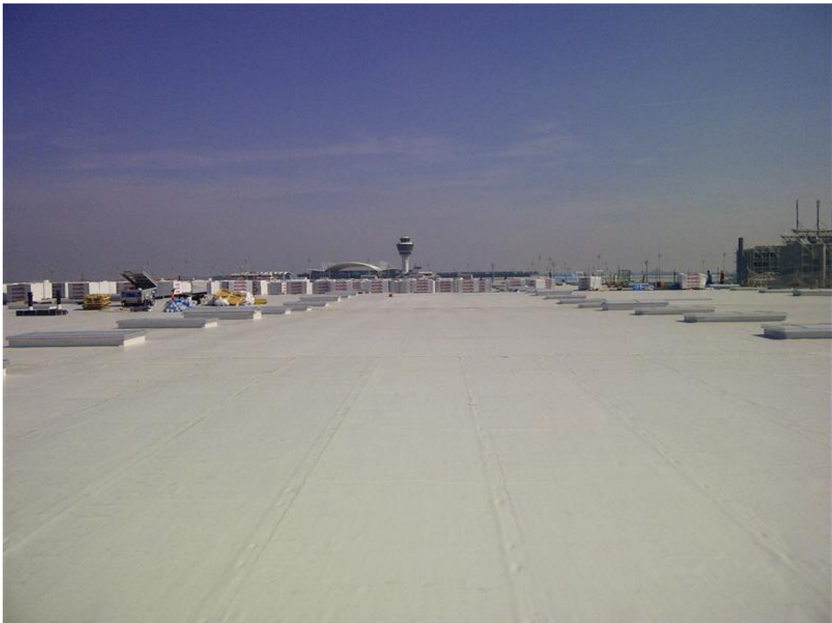
Figure 3: MAPEPLAN PLUS on fully exposed roof
