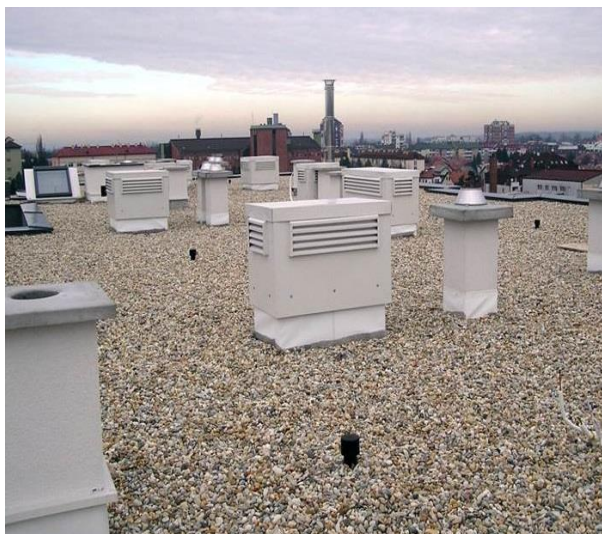
Figure 6: Installation with ballast
