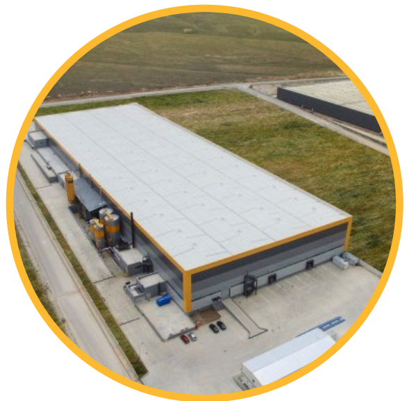
ODE Eskişehir, Turkey Production Facilities
