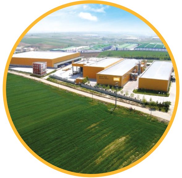
ODE Çorlu/Tekirdağ, Turkey Production Facilities
