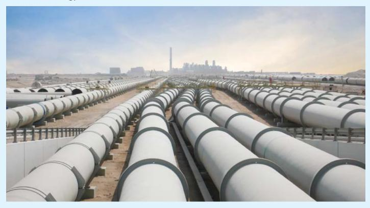
Future Pipe Industries GRP Pipes are made from glass fiber reinforcements that are embedded in cured thermosetting resin.
