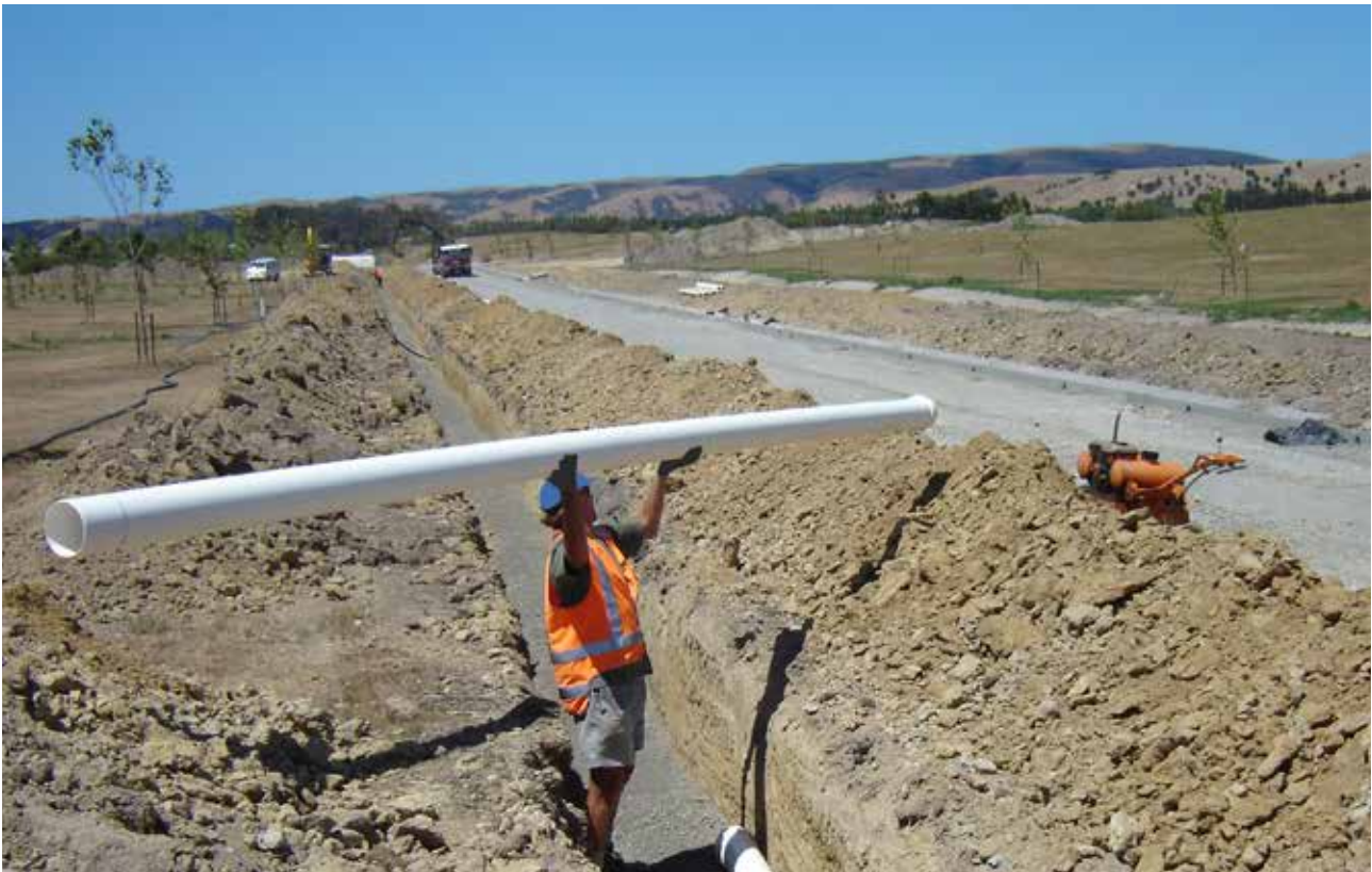
Image 1. Iplex PVC-O Pressure Pipe being installed
