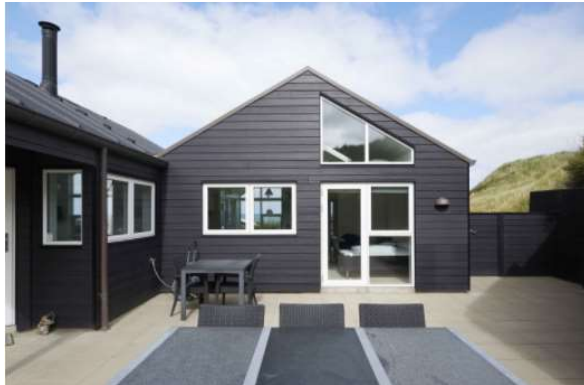
FIGURE 1: HARDIE® PLANK IN USE
