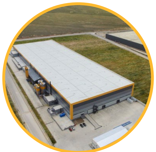
ODE Eskişehir, Turkey Production Facilities
