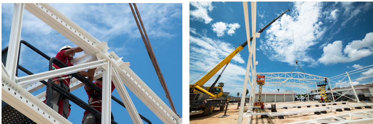
Figure 4: Installation of the Structura system
